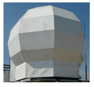
This station is designed for signals Receive in S frequency band.
