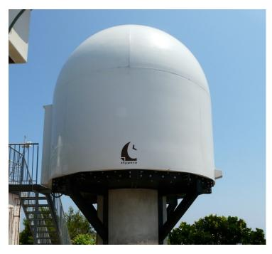
This station is designed for signals Receive in S frequency band.
